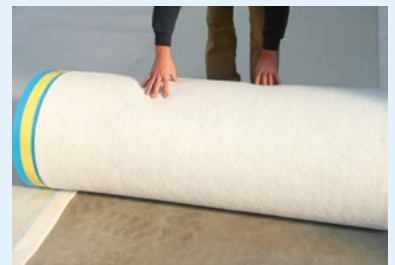
Unroll the underlay with the overlap over the lateral roll
