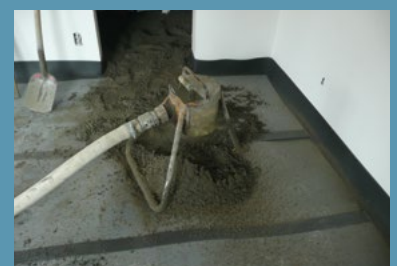
Make a \pm 8 \text{ cm} thick reinforced screed on the Bi+20
