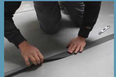
Insure the tightness with the Stickelfoam 25/70
